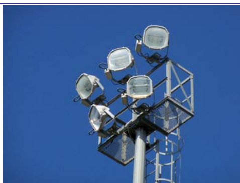
Detall focus halogenurs 2.000W torres
