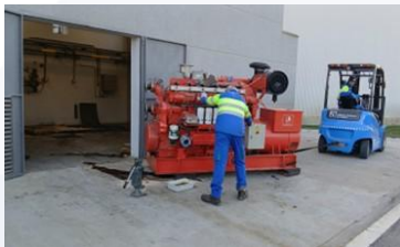
Retirada antic motor Guascor
